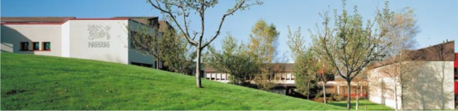
The Nestlé Research Centre located near Lausanne, Switzerland.
